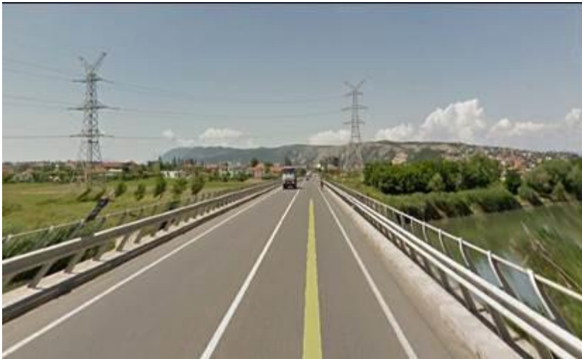
Figure 3-32 View of the existing bridge platform over Drini river in Lezhe (225 m long)
