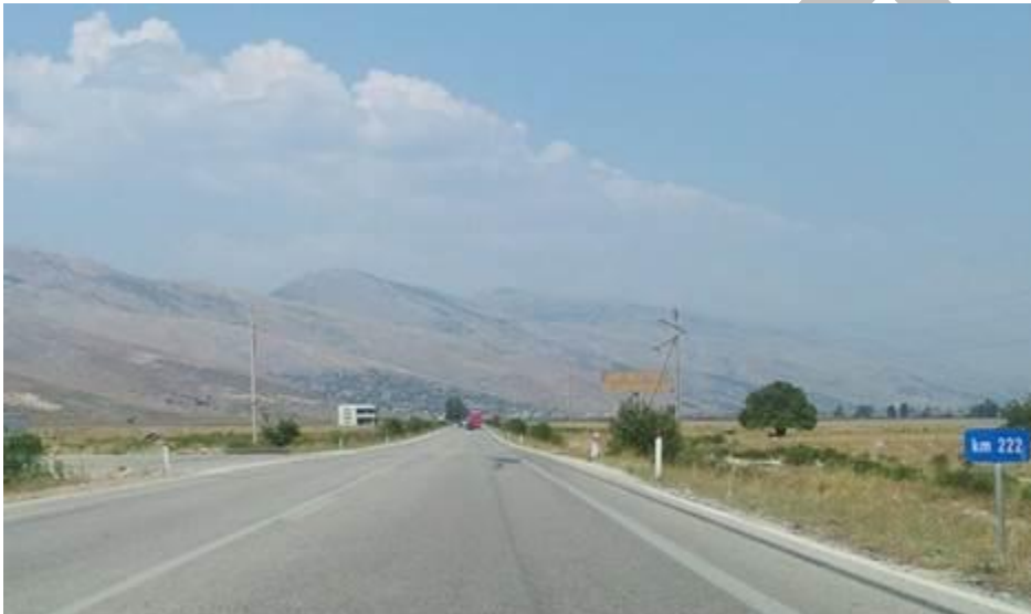
Figure 3-23 View of Section 13A
