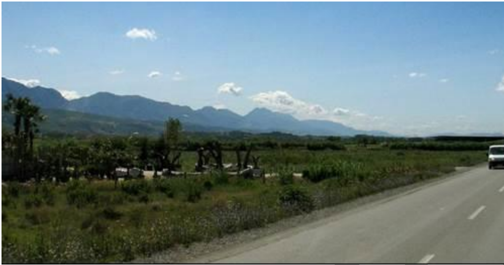
Figure 3-5 View of the second part (approx. 13.2 km) of AIC section 2
