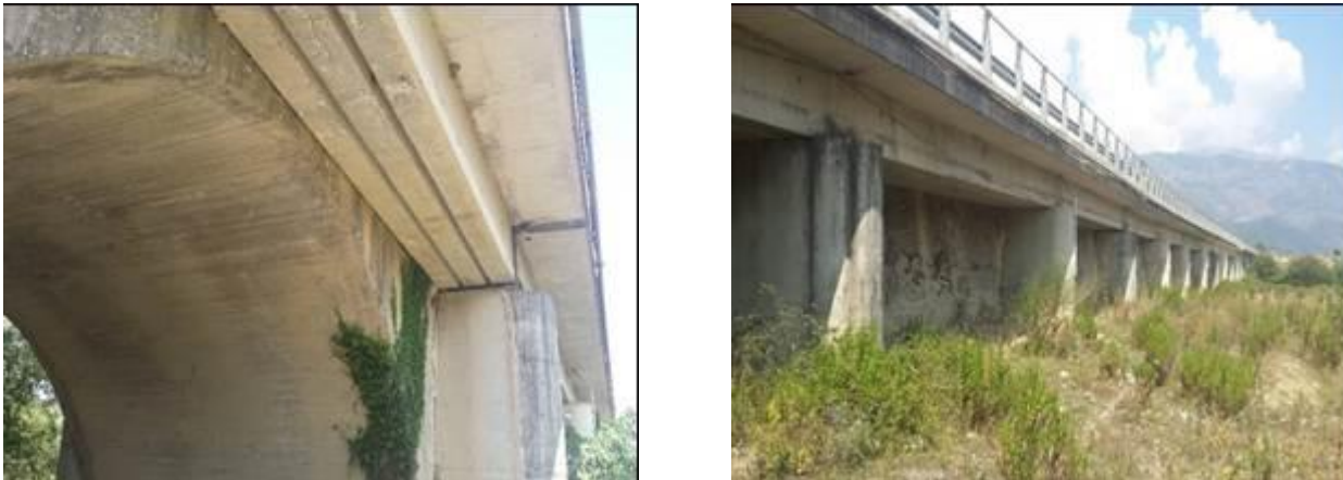
Figure 3-38 View of the existing bridge structure
