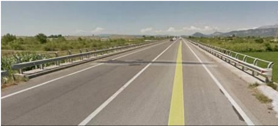
Figure 3-34 View of existing bridge platform over Mati river (625 m long)
