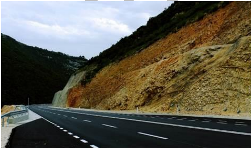
Figure 3-16 Section 9B-2 – View of the existing 1x2 lanes highway, Sh4
