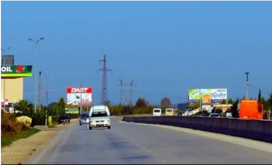
Figure 3-13 View of Section 6+7
