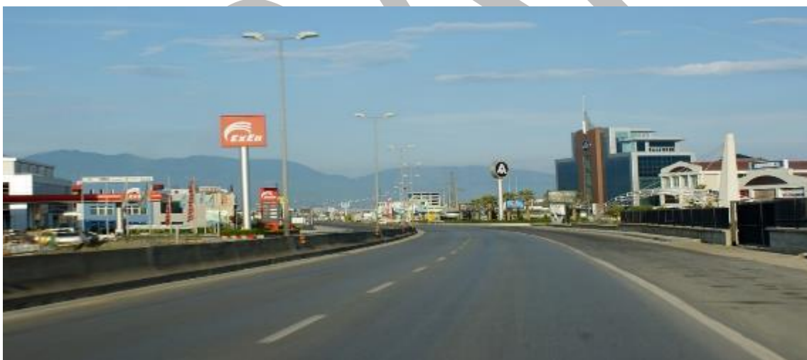
Figure 4-86 Commercial constructions along Rrogozhine Lushnje motorway
