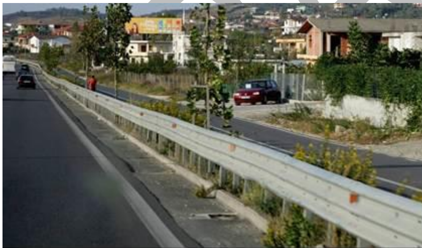
Figure 3-10 View of AIC section 5C
