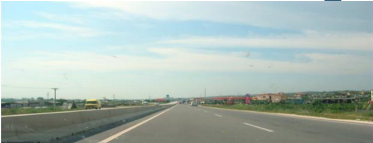
Figure 4-85 Roadsides along Sections 6 and 7
